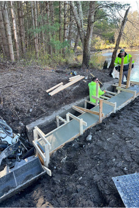
Image 12. New foundation poured.
