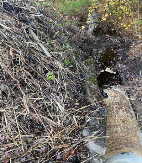
Image 9. Blockage covering area.
