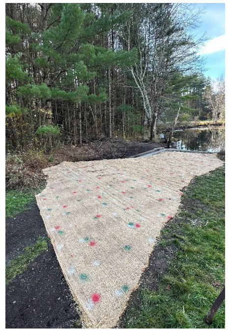
Image 14. New erosion control
