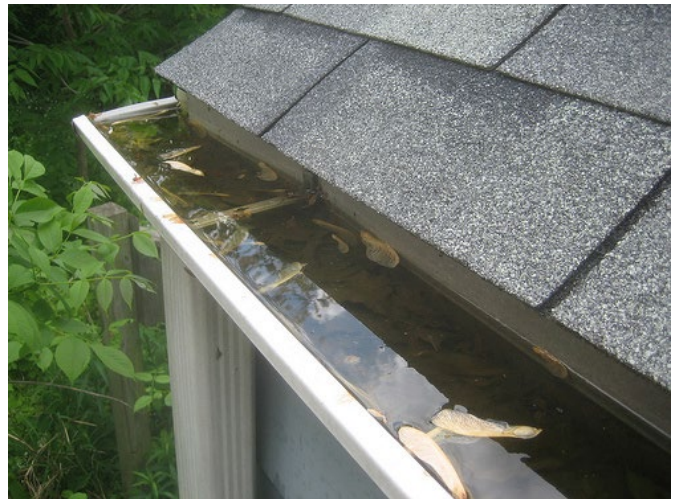
Figure 8. Clogged rain gutter filled with water
