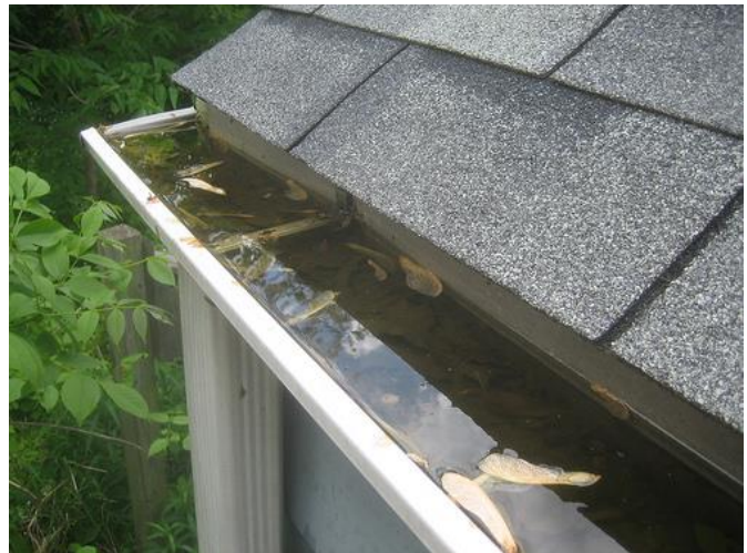
Figure 8. Clogged rain gutter filled with water
